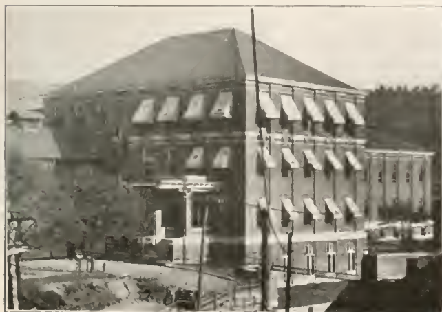
The new hospital building of the Cambria Steel Company at Johnstown, Pa. This company claims the distinction of erecting the first industrial hospital in the country.
